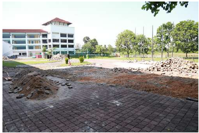
Construction of Multi purpose Court
